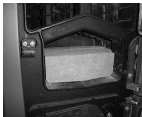
Fig. 6p. Position of ceramic catalyst on the exchanger shelves in a KLIMOSZ MULTICOMBI.
